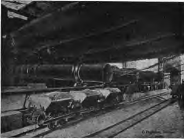
FIG. 64.—Rotary Coolers Mounted beneath Kilns.
